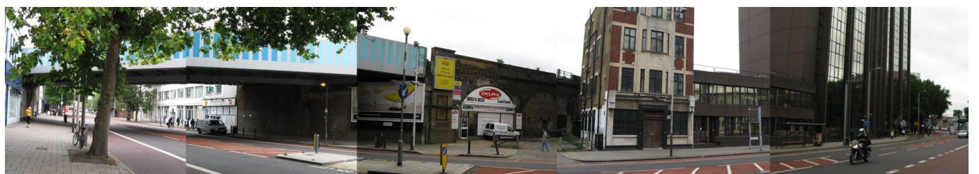
Existing street view of the Site
